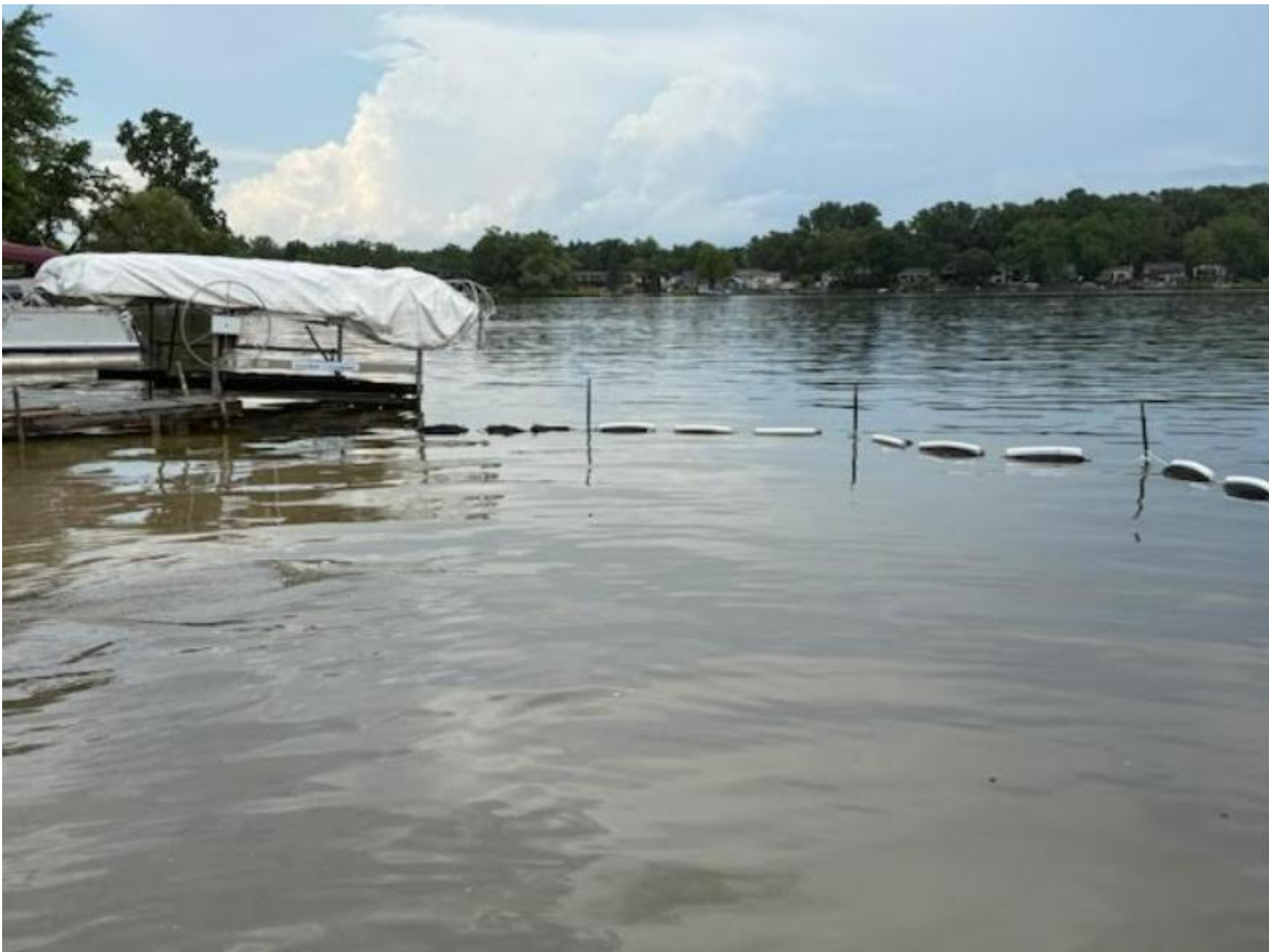
Picture 1 Of 4 at Grand River Drain outlet
